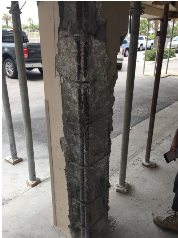
Picture 2: In-progress column demolition
