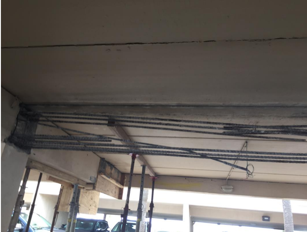
Picture 1: Demolition of the transfer beam
