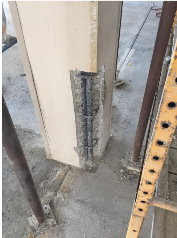
Picture 3: In-progress column demolition
