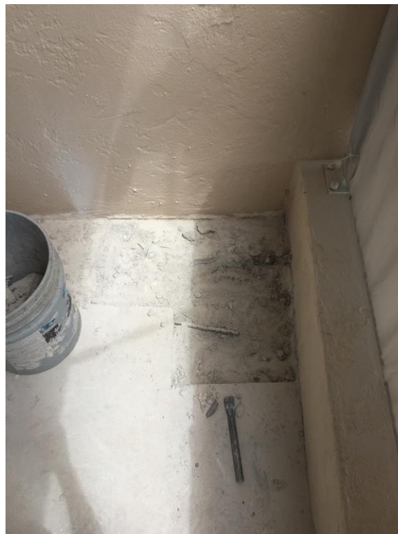
Picture 4: In-progress topside repair on 10 stack
